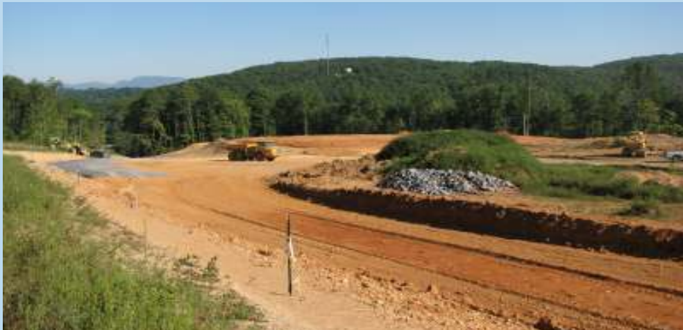
Southern Virginia University Athletic Facility Construction
